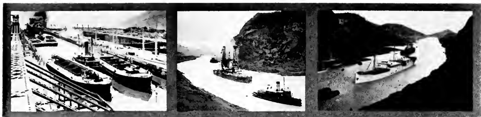
Fig. 3, left, the dredger fleet in one of the lower locks at Gatun. Fig. 8, center, the battleship "Ohio" passing Cucarache slide (this is the narrowest and most winding part of the canal). Fig. 13, right, the motorship "Jutlandia" passing through the canal in January 1915. The vessel is opposite Gold Hill.
